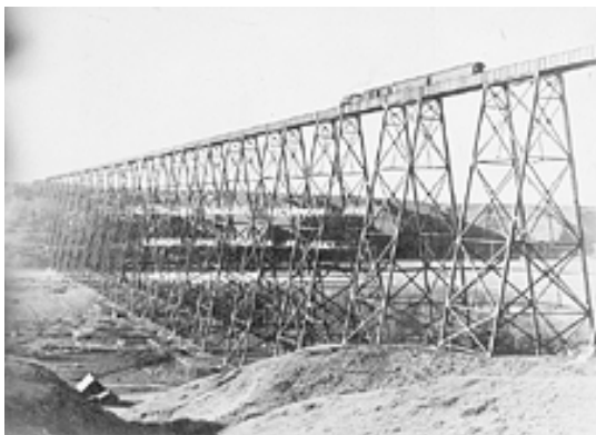
27. Lethbridge Viaduct, Alberta
