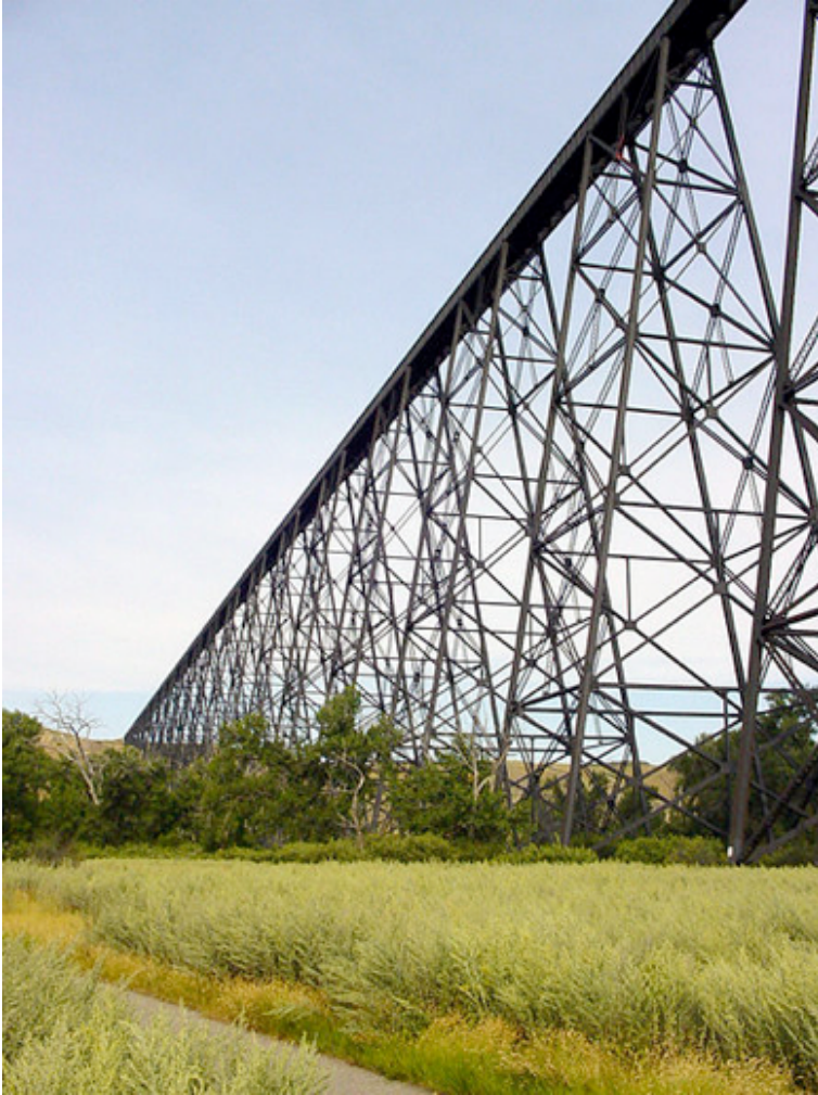
28. Lethbridge Viaduct, Alberta
